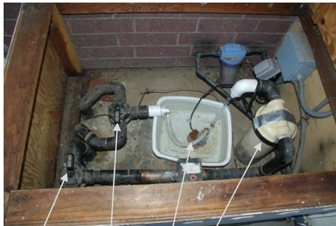
Valve A Valve B Pump Filter Figure 4
