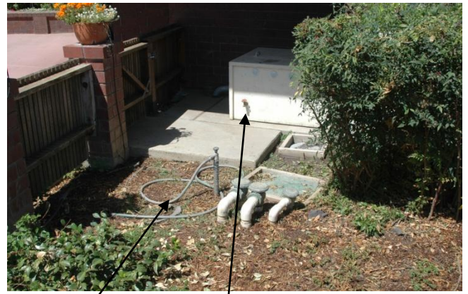
Hose to connect to faucet when Figure 9 draining font. Use hose to keep water off concrete pad.
